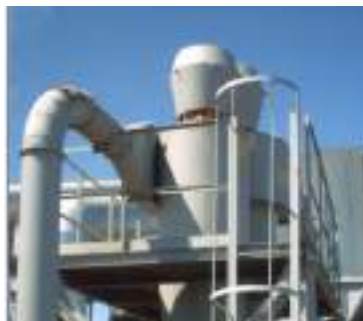
Fig.3. Source of 322 Hz frequency measured outside on the roof of production shop, with resonance of the cyclone construction.
